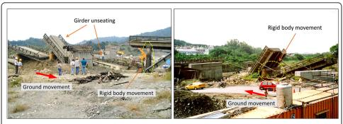
**Fig. 13** The collapsed spans of the E-Jian Bridge due to surface faulting movement. Images are modified from Lee and Loh (2000)
