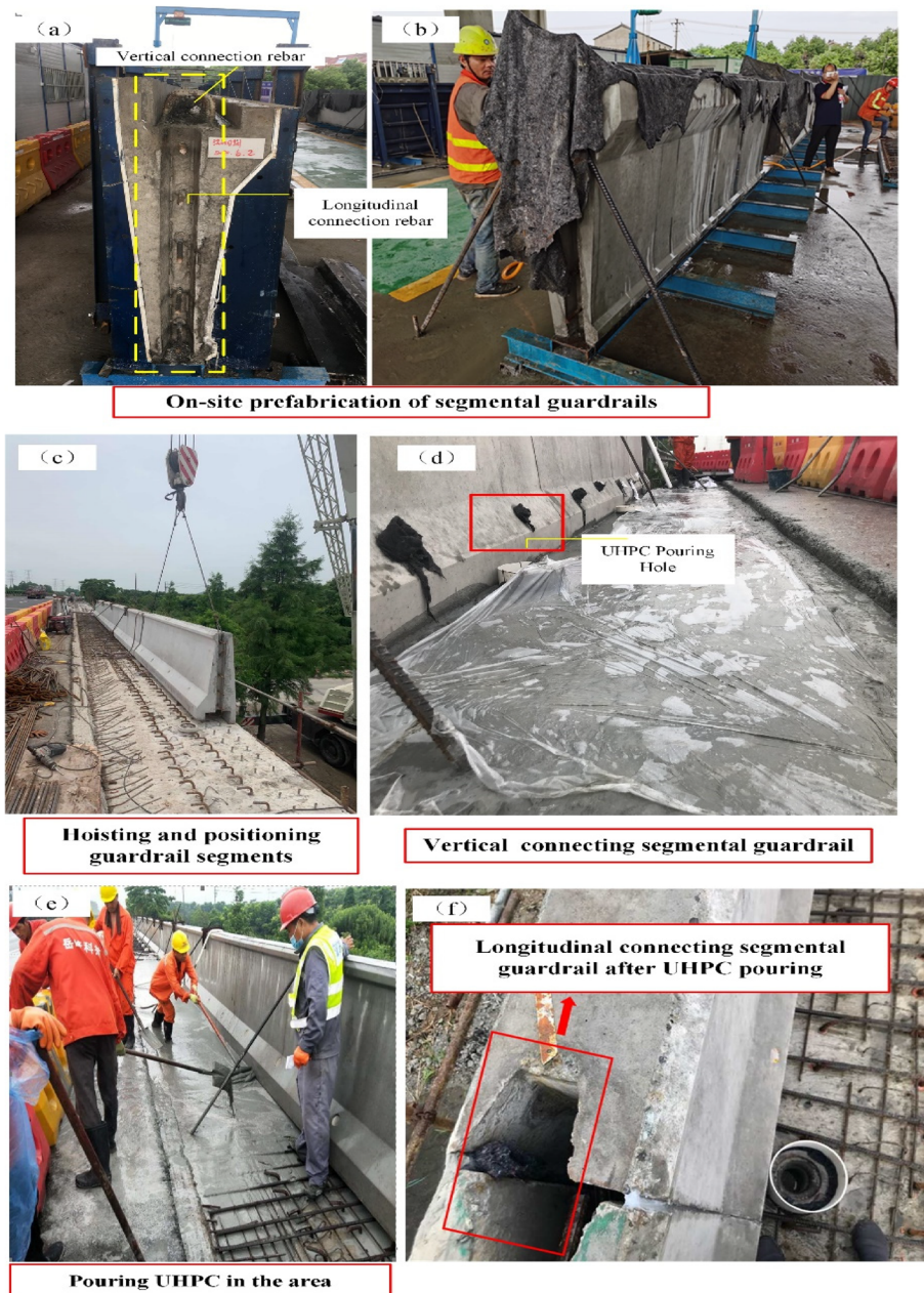
Fig. 20 Main process of existing bridge guardrail reconstruction
