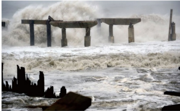
Fig. 1 Collapse of sea-crossing bridges
