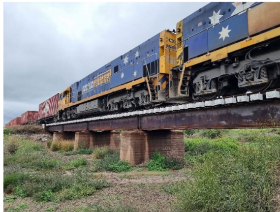
Fig. 7 Train 3SP7 passing over the bridge
