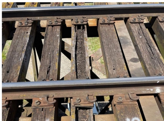
Fig. 1 Example of timber transoms in a bridge in very different conditions from fair to very poor
