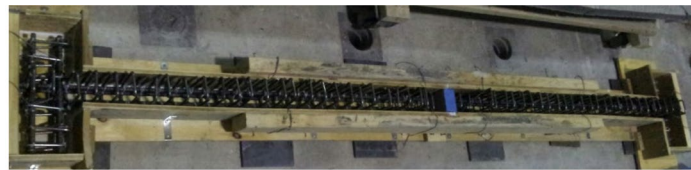
(c) Girder reinforcement and formwork
