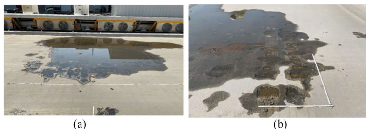
Fig. 8 Visual inspection images from the inspection reports of the testbed (a) Small to large spalls looking east 3,25 m 2 (35 sq.ft.); (b) large spalls looking south 2,32 m 2 (25 sq.ft.)
