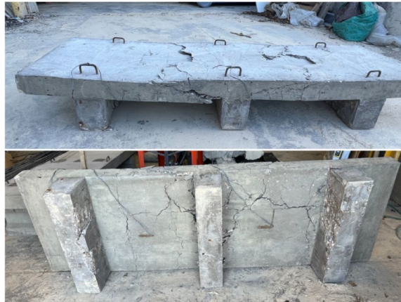
Fig. 14 RC Decks Failure Mode, and Cracks
