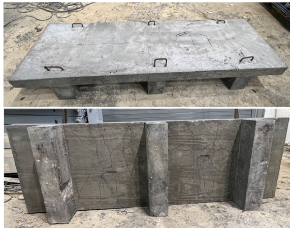
Fig. 15 SFRC Decks Failure Mode, and Cracks
