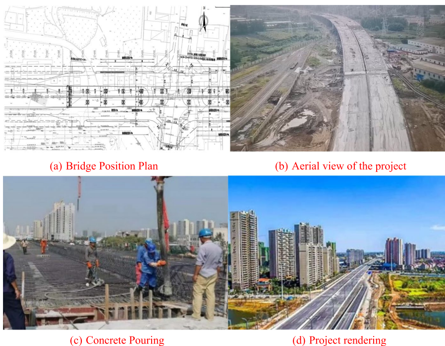
Fig. 7 Jingzhou Xingang Avenue cross-line bridge project
