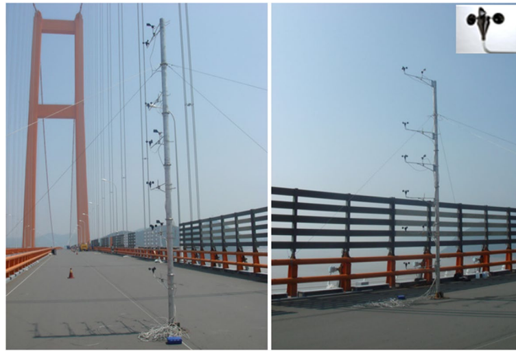
Fig. 10 Field measurement of wind environment on bridge deck
